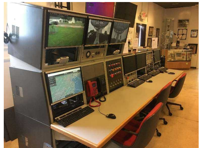
Figure 18- ISEC Control Center
