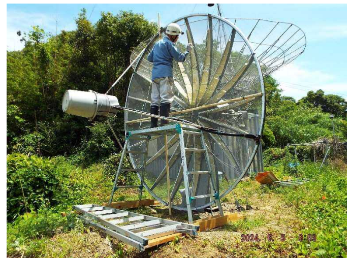
Figure 30 - JA6AHB dish repair
