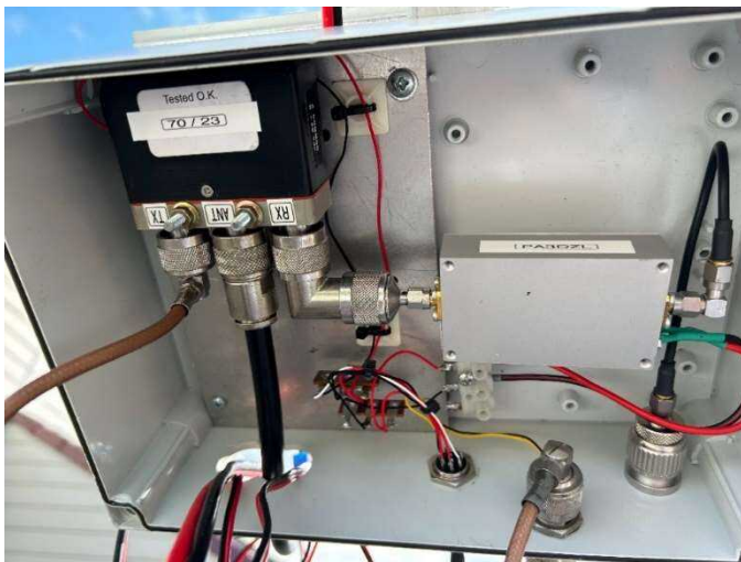
Figure 28 - PA3DZL N coax switch + preamp
