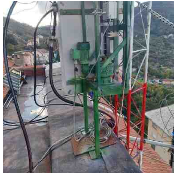
IK1FJI tower strengthening
